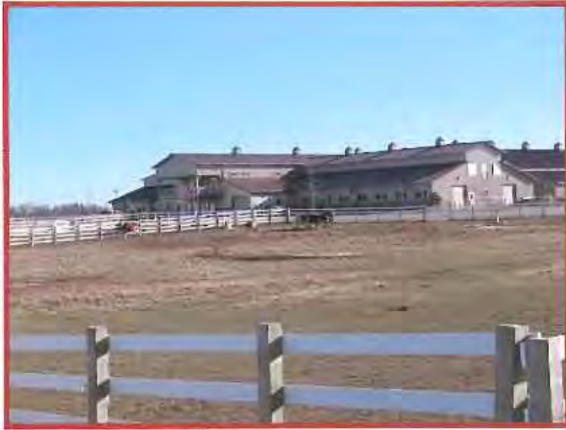
Figure #8. The Minnesota Equestrian Center situated at junction of County Roads 21 and 44. The Equestrian Center is a nationally recognized facility serving the needs of horse owners and enthusiasts alike.
